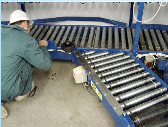
Installation of the roller track conveyor system.
